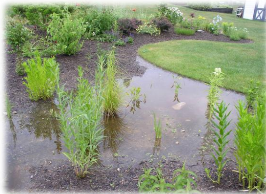
The native plants in this rain garden are working hard to capture, filter, and slowly release the recent rains.
